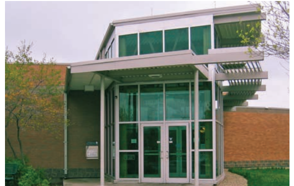
A view of the main entrance of the Alice Turner Branch Library. Deciduous trees to the south block unwanted summer solar heat gain. Conifer trees to the north protect the building from prevailing winter winds.
