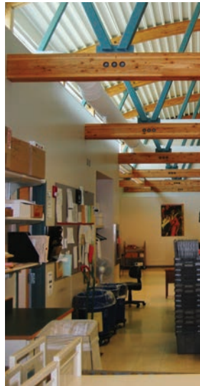
View of the clerestory windows bringing daylight into the back offices.
